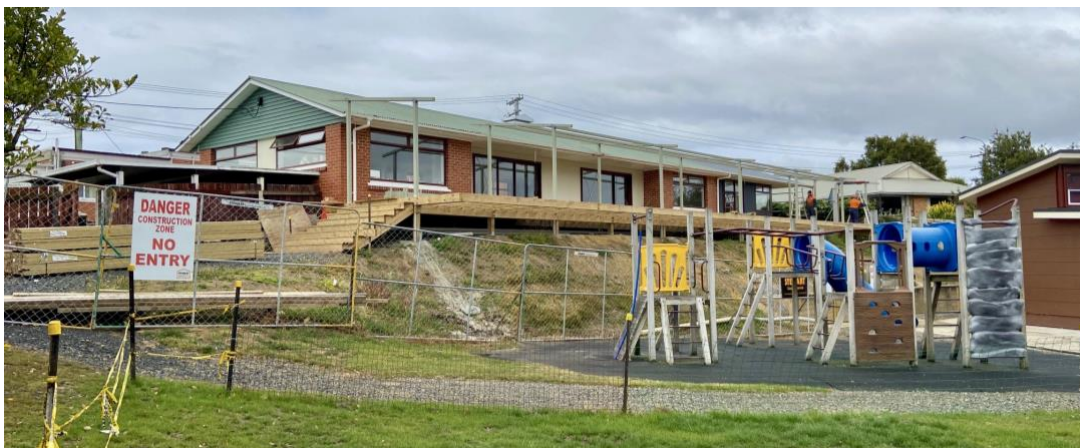
ABOVE: Our new classrooms are coming along on schedule!
